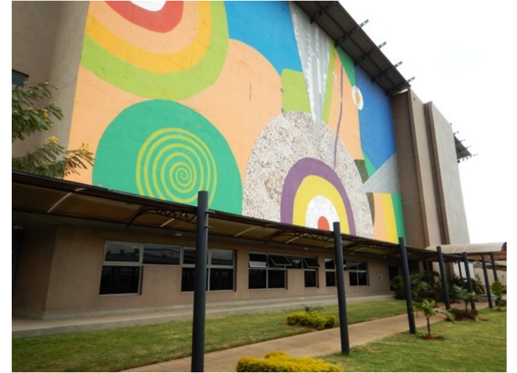
Data Centre, Nairobi, 2015
